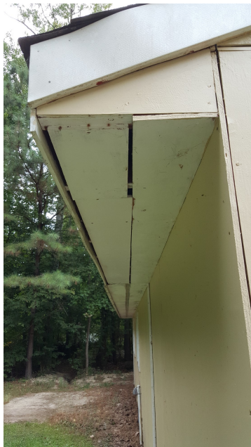
Soffit needs repair
