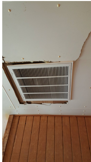
Wall around ac/heating vent needs repair
